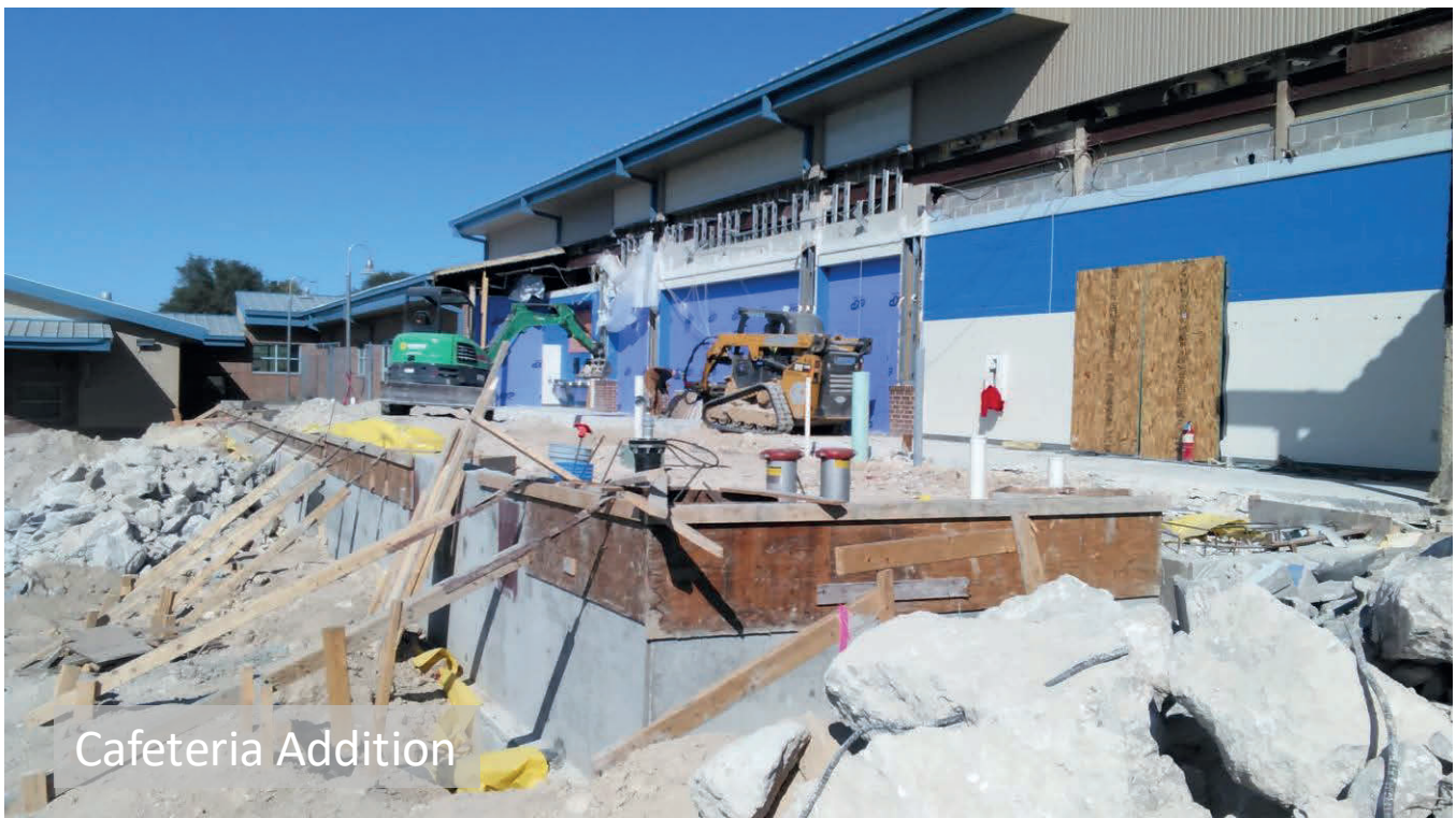
Two Story Classroom Addition
